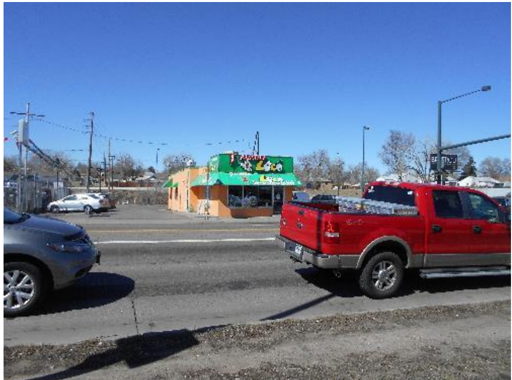
22. View of 775 Federal Boulevard (El Cameron Loco Restaurant) facing west from the western side of Federal Boulevard.
